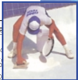
Step 1 Pool Preparation
