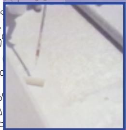
Step 4 Fiberglass Mat
