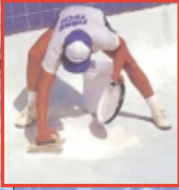
Step 1: Pool Preparation
