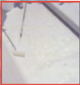
Step 4: Fiberglass Mat
